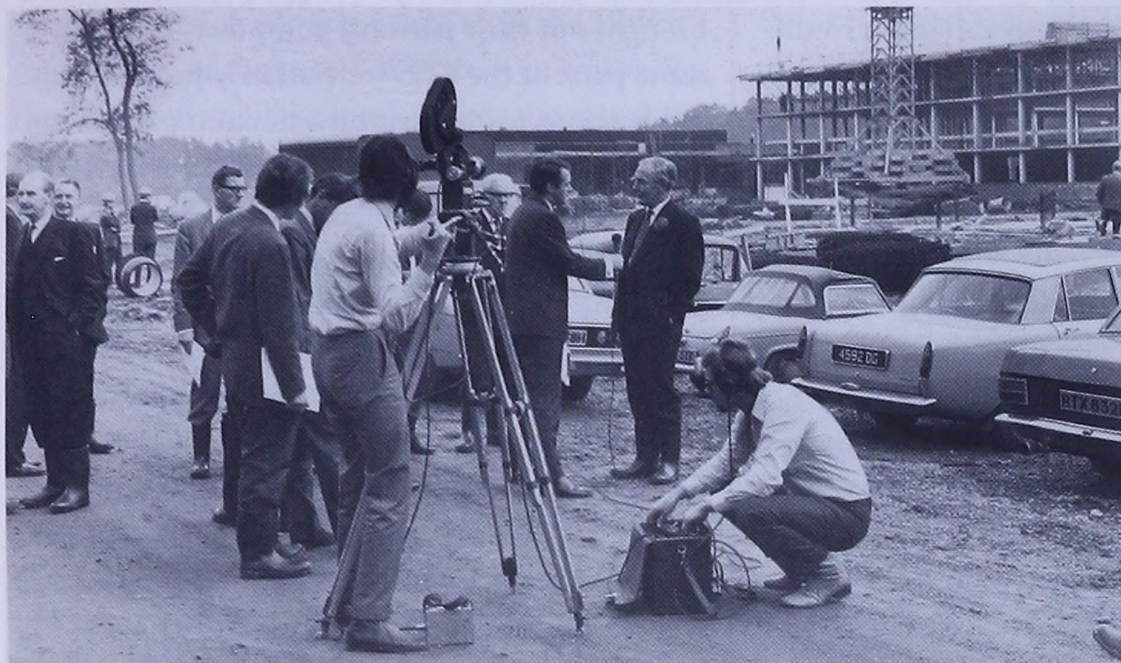
Construction of the Business Statistics Office, Newport - October 1970
